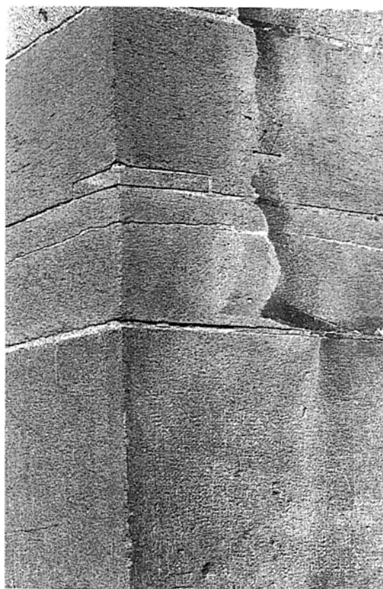
Figure 8: Very sound greenschist ashlars on a pillar of the south chapel of the Nidaros cathedral. The pillar have been slightly redressed (1872). Note the preserved mason's mark from 1180-90.
