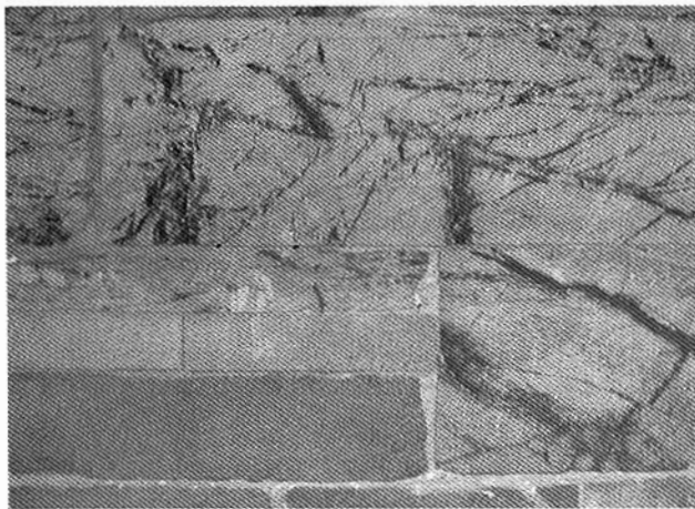
Fig. 4 – Klungen-like stone at Nidaros Cathedral. Note dark oxidised veins of carbonate minerals. Photo: Storemyr 2000.
