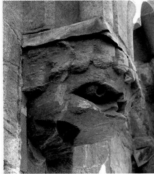
Fig. 5 Medieval head made of Klungen stone at Nidaros Cathedral. Note that the lower part is broken along a foliation plane. Photo: Storemyr 2000.
