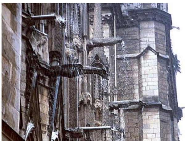
Figure 4. Gargoyles getting rid of water during a heavy downpour at Notre Dame in Paris
